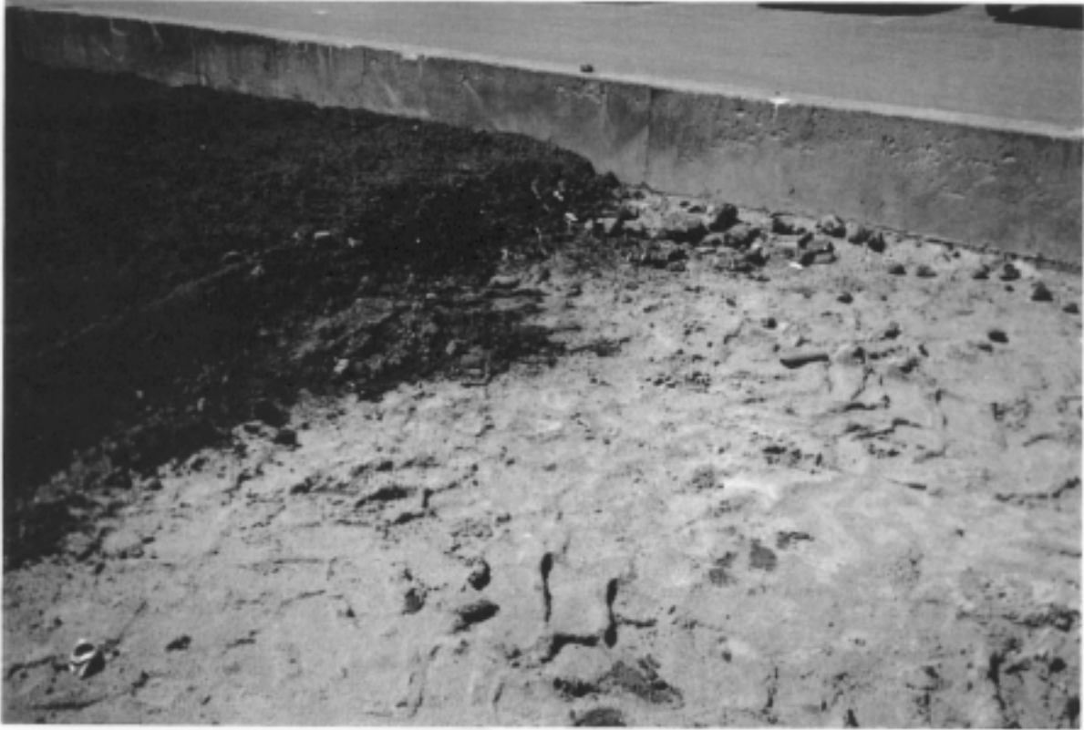
Photo 2: Placement of top soil over sand fill base.
